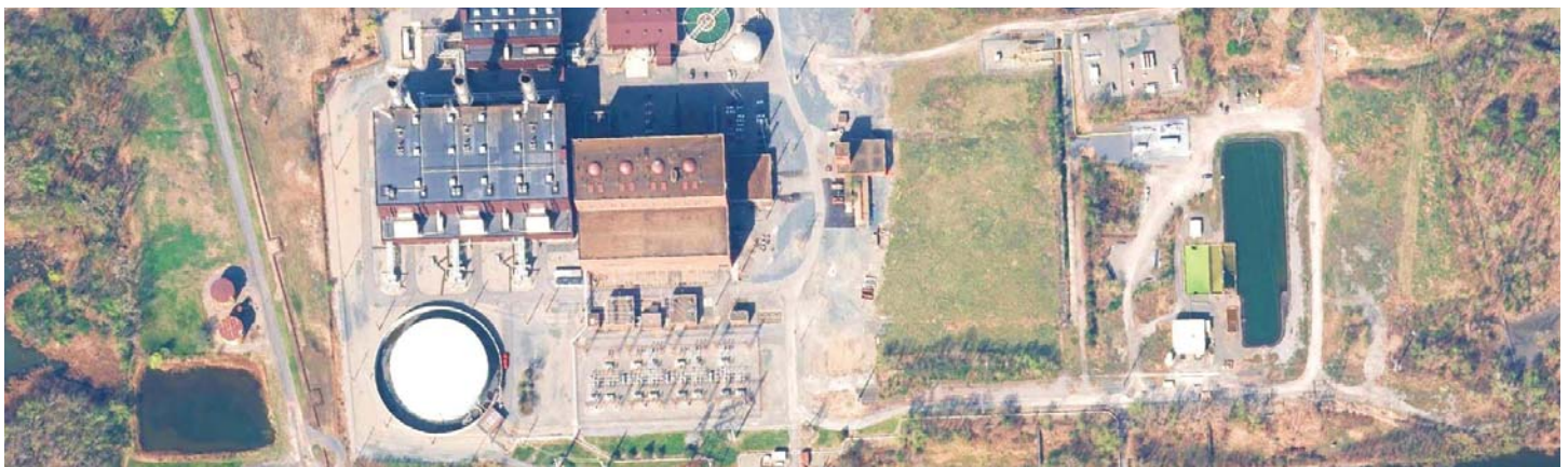
BETHLEHEM ENERGY CENTER
