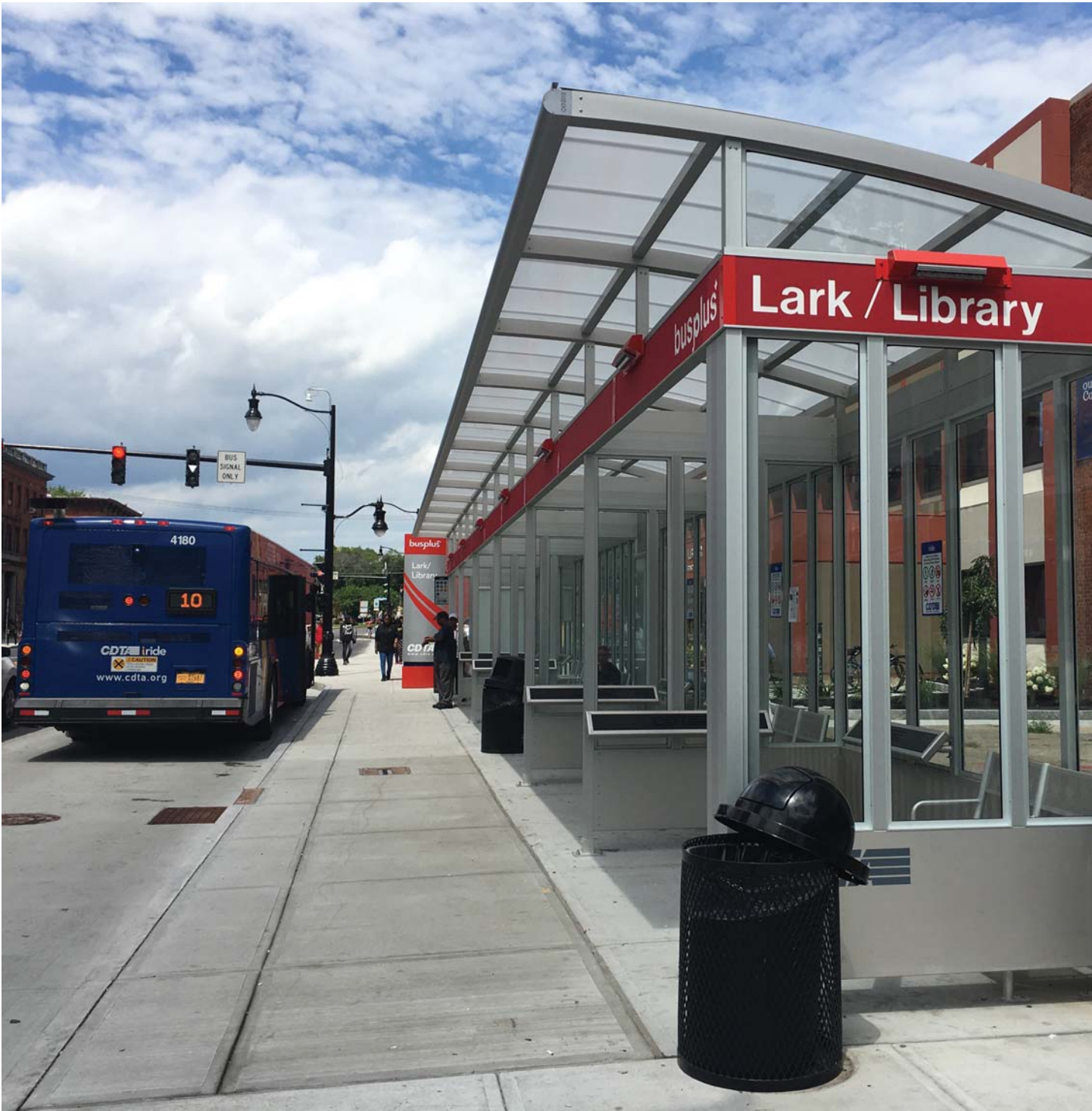
Recently renovated CDTA bus stop in downtown Albany.
