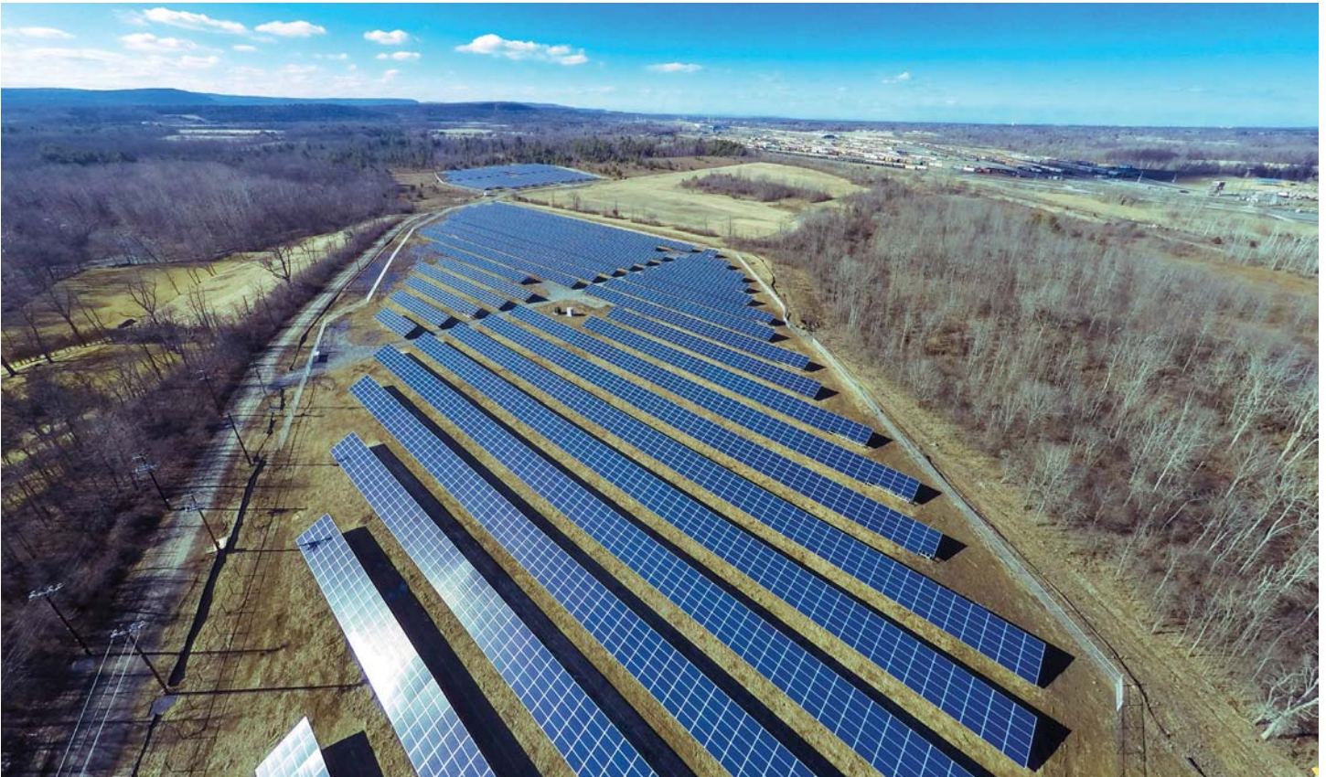
Solar Arrays in Albany County. The top image shows the Capital Region Community Solar Garden in Altamont, which came online in April 2019. The bottom image displays the Bethlehem East solar farm, which was developed on a former clay mine site and supplies town facilities with electricity. Photo credits: Solar Industry Magazine (top image); NextEra Energy Resources (bottom image).
